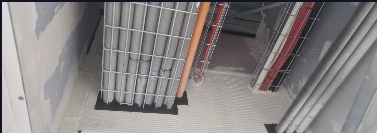
■ Firestopped service penetrations, sealed and recorded before cover-up.
